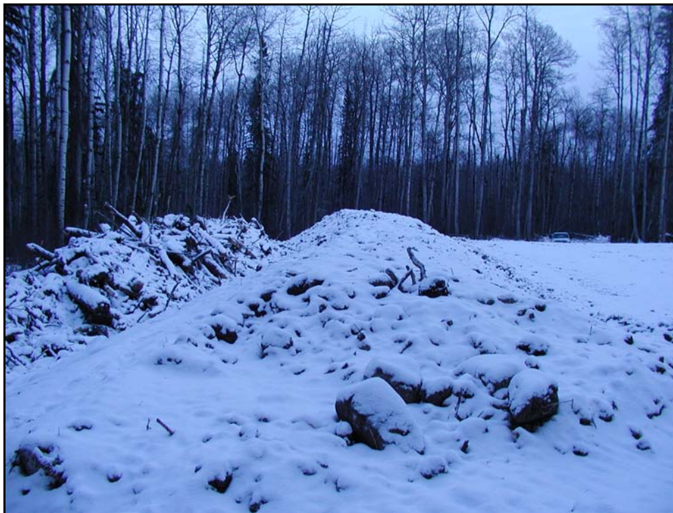
Fig. 3.6. Separate slash pile and rooting zone pile with mineral subsoil used to level lease. (photo: Terry Osko)
