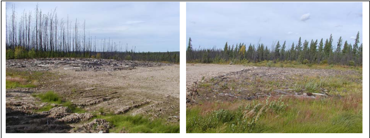
Fig. 7.2. An OSE located near the edge of a small upland ridge within a predominantly lowland area. The lease was constructed by transferring the upslope mineral material down slope to produce a level pad and then moving the material back upslope upon abandonment. The result is a disturbed upslope position and a buried down slope position due to incomplete removal of transferred materials. Moving the well centre approximately 40 m to a level location would have reduced construction costs and footprint intensity by eliminating the need for any soil disturbance at all. (photos: Terry Osko)
