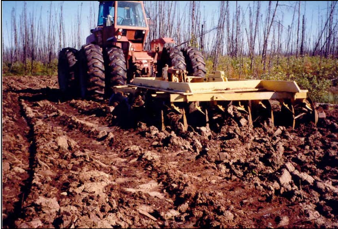
Fig. 6.1. Disking to loosen soil surface on clay pad constructed for an observation well related to a Steam Assisted Gravity Drainage pilot. In this case, salvaged peat was also incorporated into the soil with the disk. (photo: Barb Thomas)
