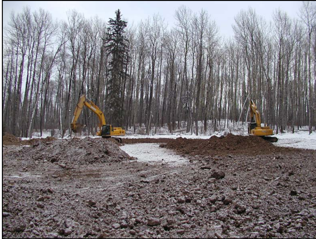
Fig. 3.7. Progressive replacement of rooting zone with 2 trackhoes. (photo: Terry Osko)
